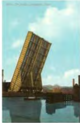
Roller Lift Bridge, Bridgeport, Connecticut - 22hx14w-Artprint
