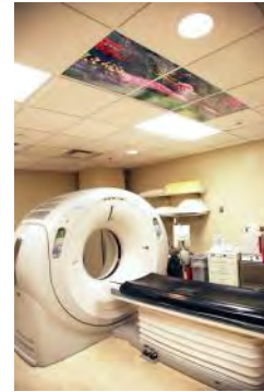
63- St. Joseph CT Room 2' x 6' UNLIT Ceiling Panel-Installation
